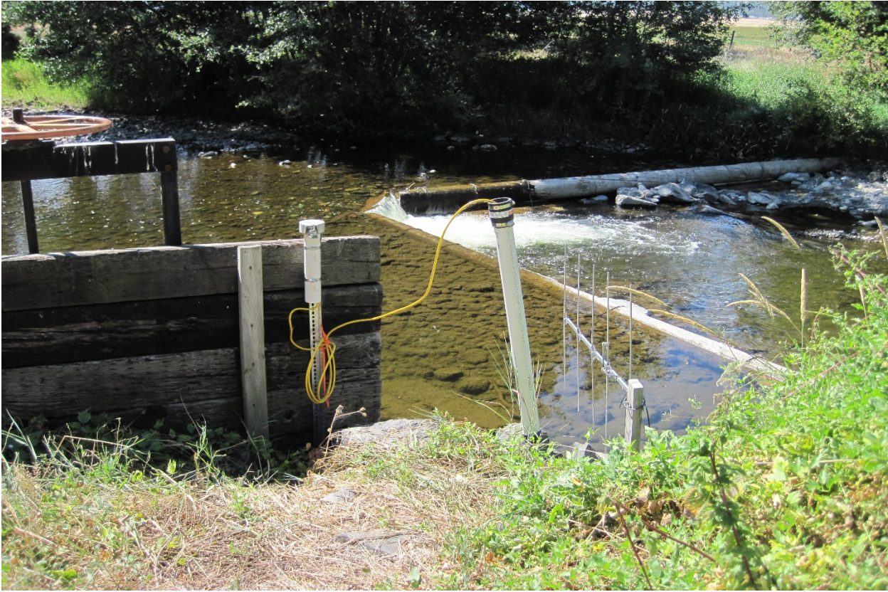
Photo point #5: Before (top) and after (bottom)
