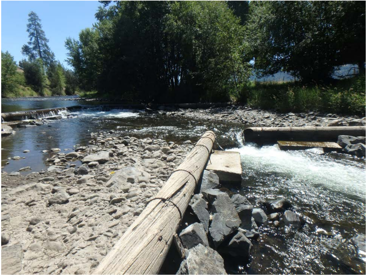
Figure 1. Photo taken below two log weirs downstream of the headgate, August 4, 2016.
