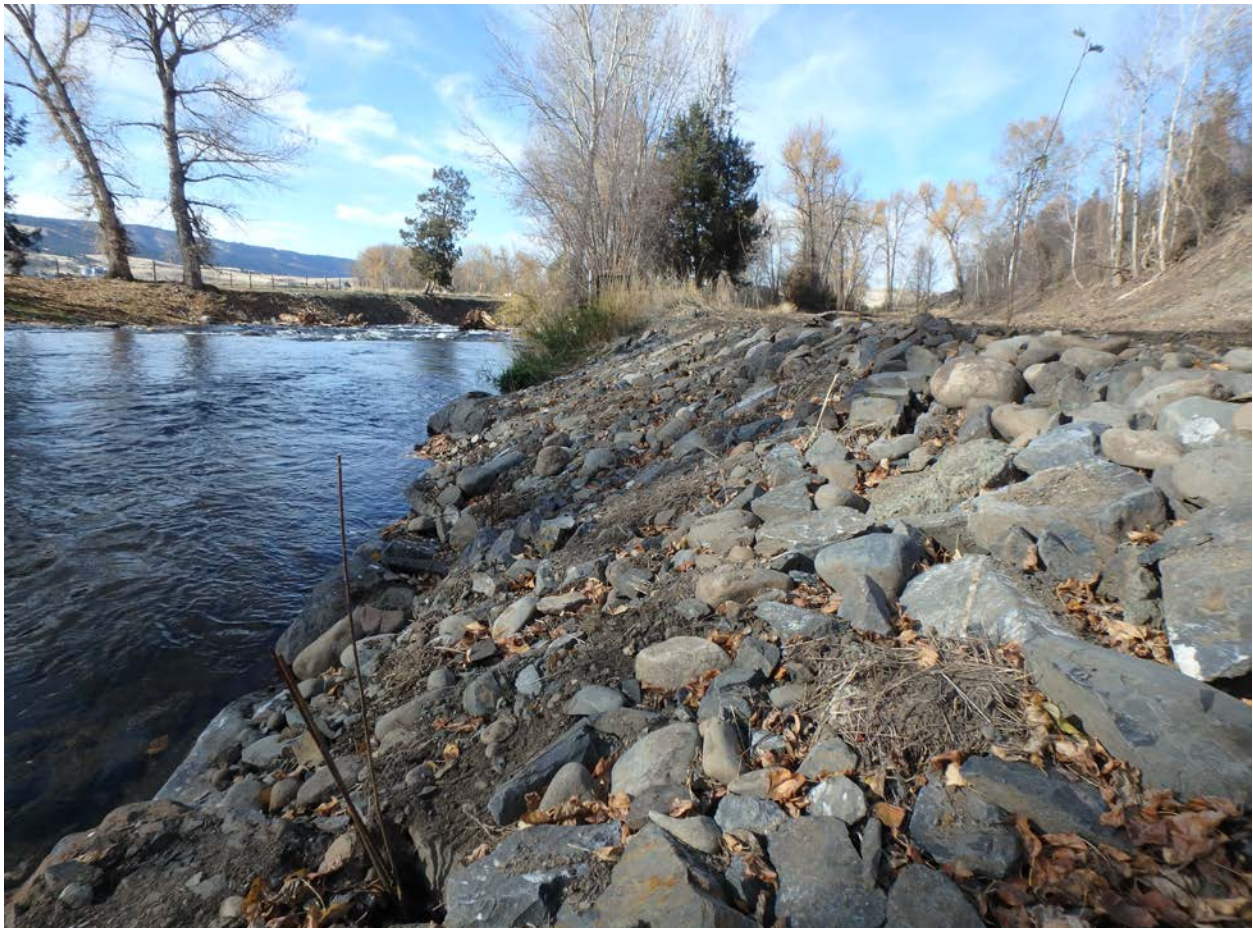
Figure 6. Willow whips were planted in the bank and container plants of various native trees and shrubs were planted on the floodplain bench throughout the project reach.
