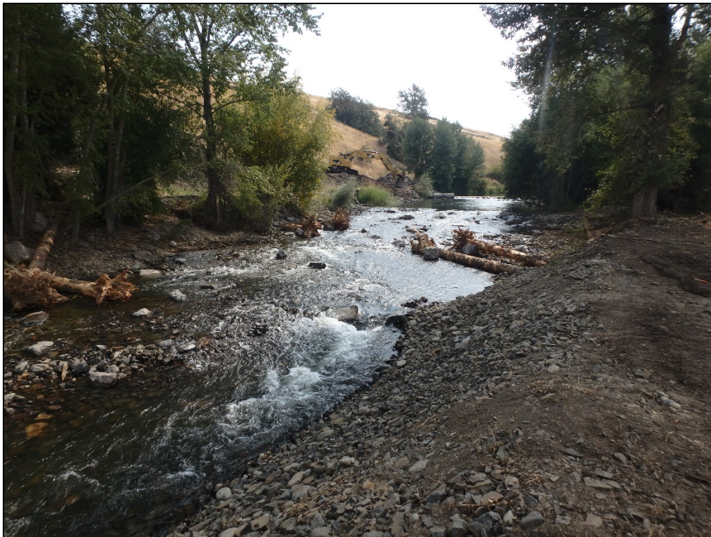
Photo 13. October 4, 2017 photo point #4 (before) from river left looking upstream, mid-project.
