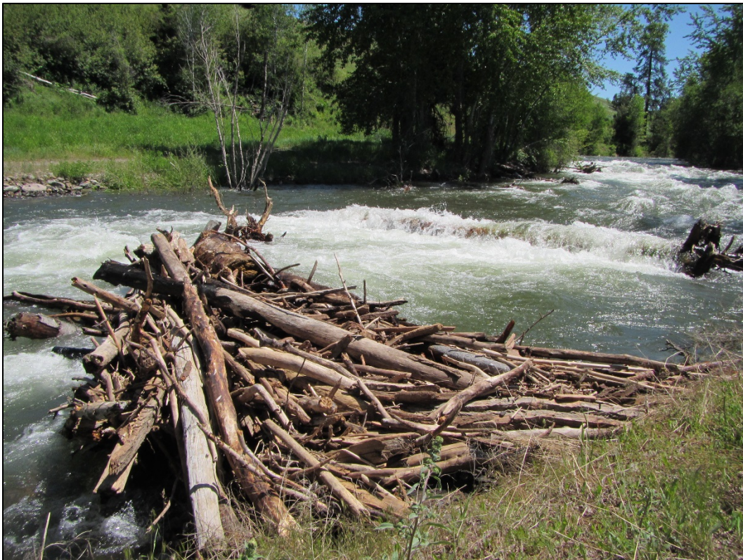
Photo 2. Photo taken June 4, 2019 showing increased size of second and third large wood structures on river left due to naturally occurring racking.
