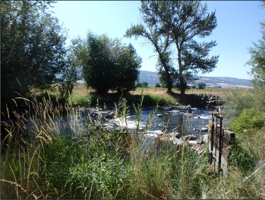
Photo 5. August 28, 2019 photo point #1, 2-years post project completion.
