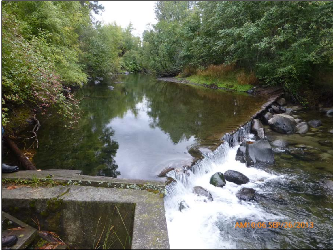
Photo 3: The wooden point of diversion effectively diverts water but as flow declines aquatic organism passage declines. Flow at the time of the photos was 40 cfs and as flow drop to approximately 20 cfs or less migrating Chinook salmon cannot get past this structure.
