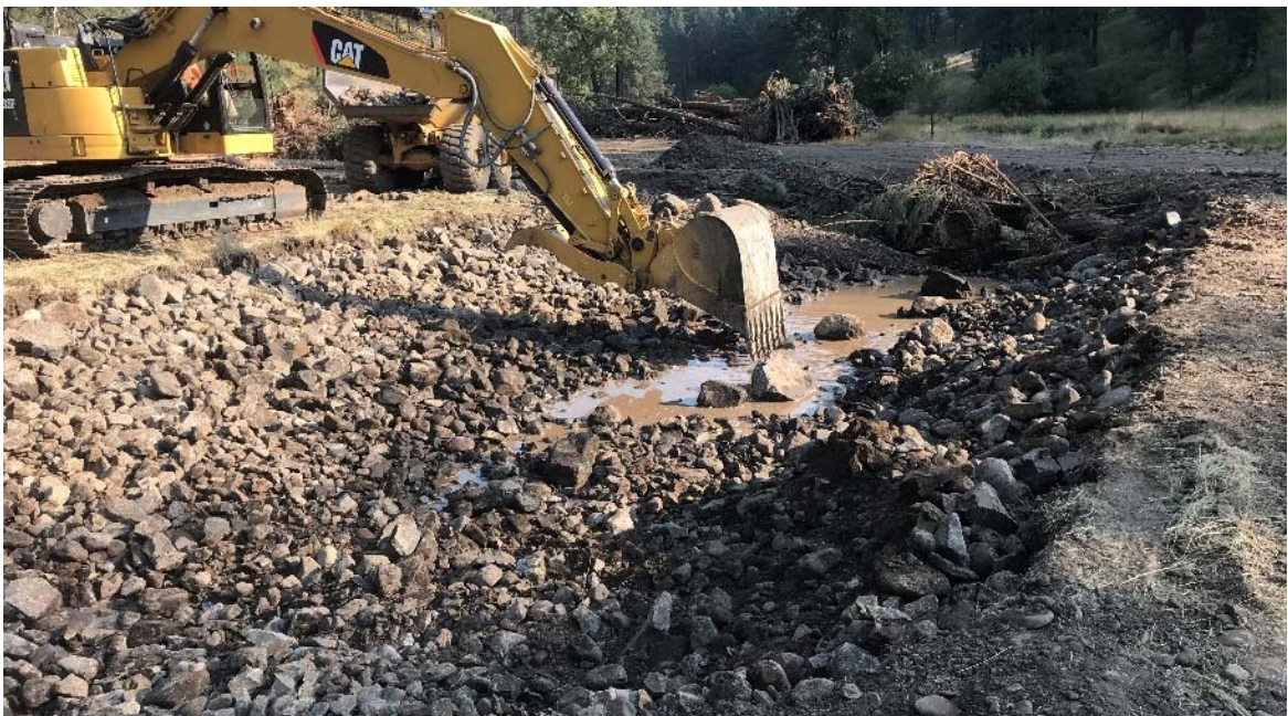
Riffle Construction and Boulder Placement
