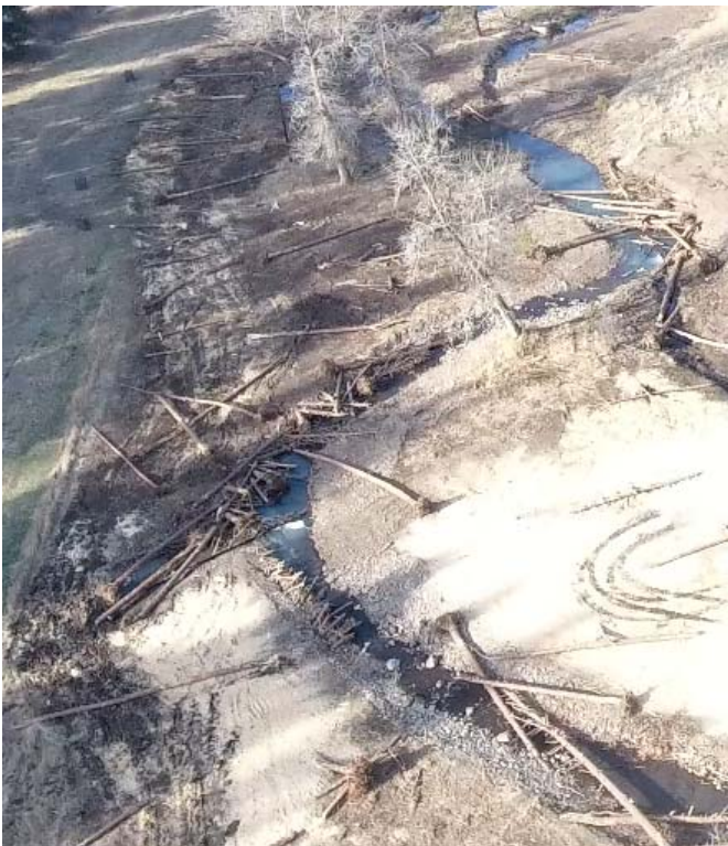
Type 2 Large Wood Structure
