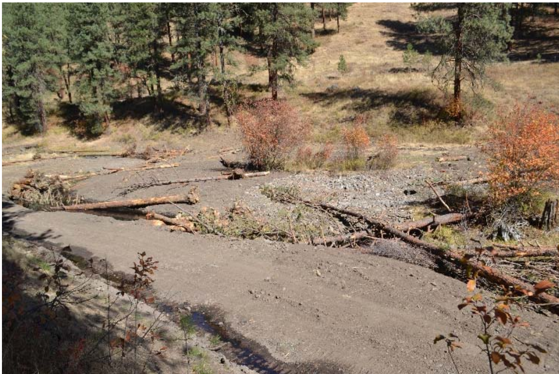
During project construction-- new channel alignment with added large wood.
