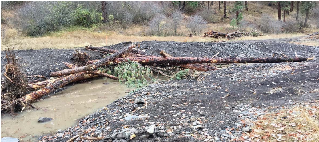
Type 2 Large Wood Structure
