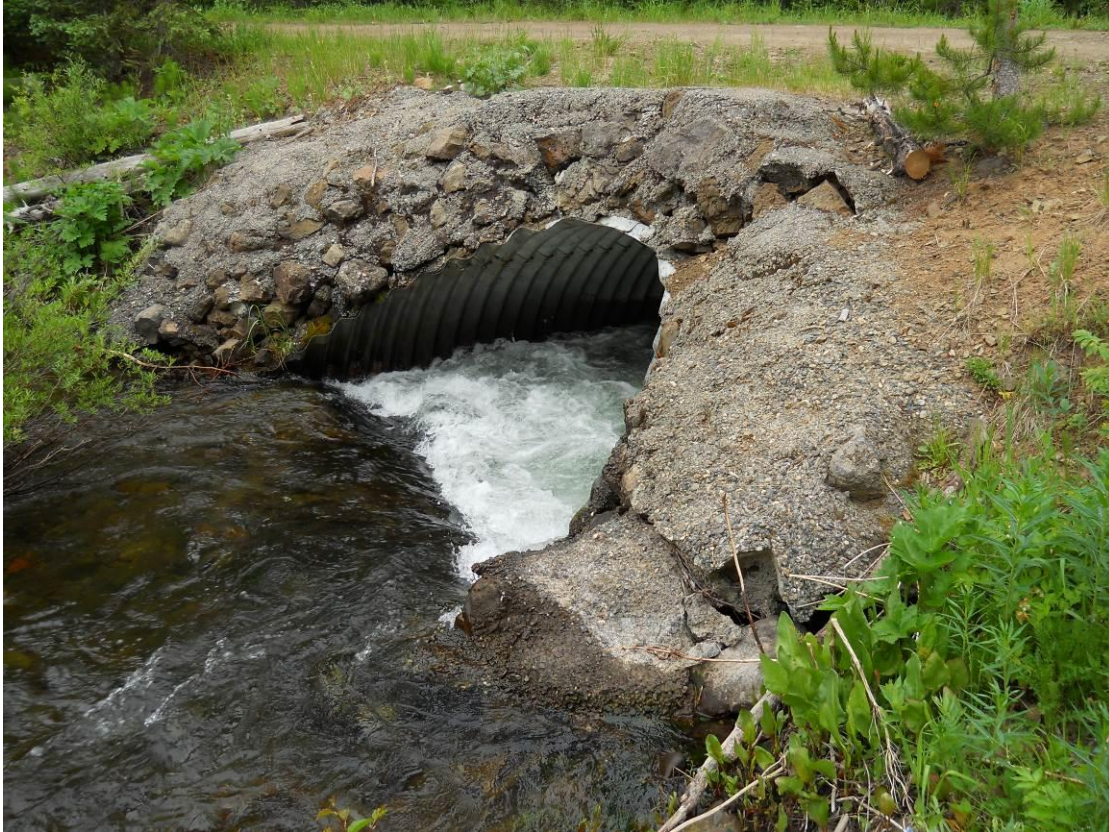
Figure 2. Lick Creek Culvert, upstream view (2011).
