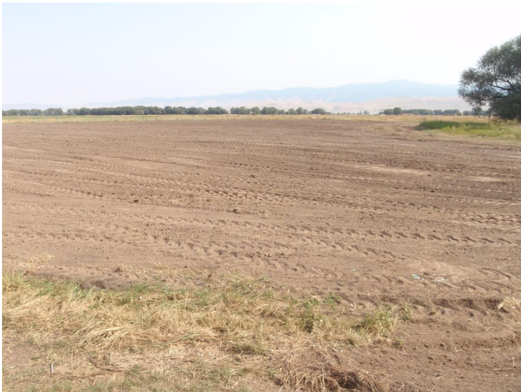
Photo 20. Completed excavated soils material leveled, mulched, and re-seeded on pasture.
