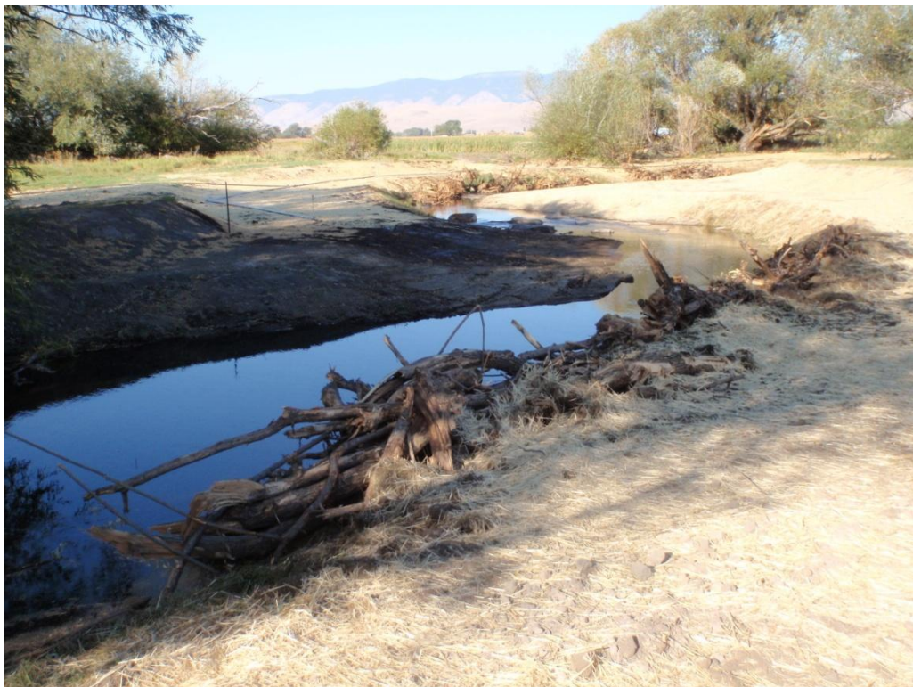
Photo 12. New meander. Excavated and re-sloped (3:1) vertical banks and widened floodplain. Large wood structures and racking materials placement. Banks were mulched, re-seeded, and planted with whips, container plants and protected with panel pods.
