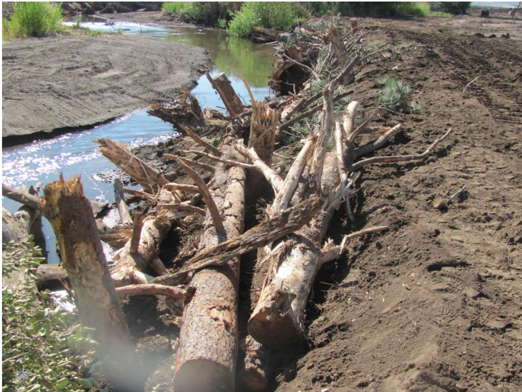
Photo 9. Typical large wood structure and racking material placement throughout project area.
