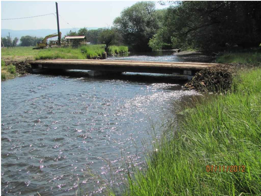
Photo 21. Temporary bridge crossing for construction equipment, protecting valuable fish habitat and passage.
