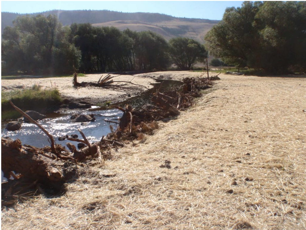
Photo 7. Upstream end of new meander. Excavated and re-sloped (3:1) vertical banks and widened floodplain. In-stream boulders, large wood structures, racking materials, and sedge mat placement. Banks were re-seeded, mulched, and planted with whips, container plants, and protected with panel pods.
