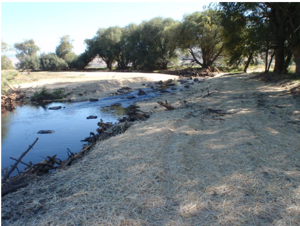
Photo 8. Downstream end of new meander. Excavated and re-sloped (3:1) vertical banks and widened floodplain. In-stream boulders, large wood structures, racking materials, and sedge mat placement. Banks were re-seeded, mulched, and planted with whips, container plants, and protected with panel pods.
