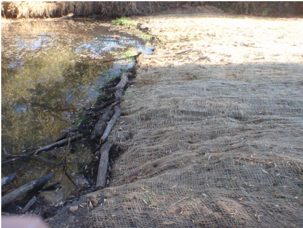
Photo 18. High water alcove with erosion control blanket, re-seeded, mulched, re-planted with whips, container plants, and protected with panel pods.
