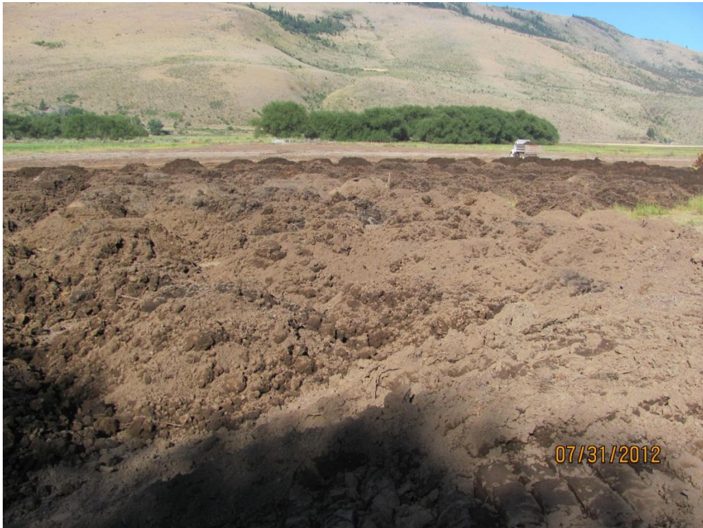
Photo 19. Excavated spoils material placed on pasture.
