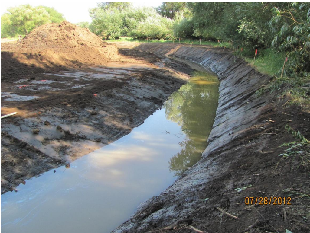
Photo 6. Excavation of new meander.
