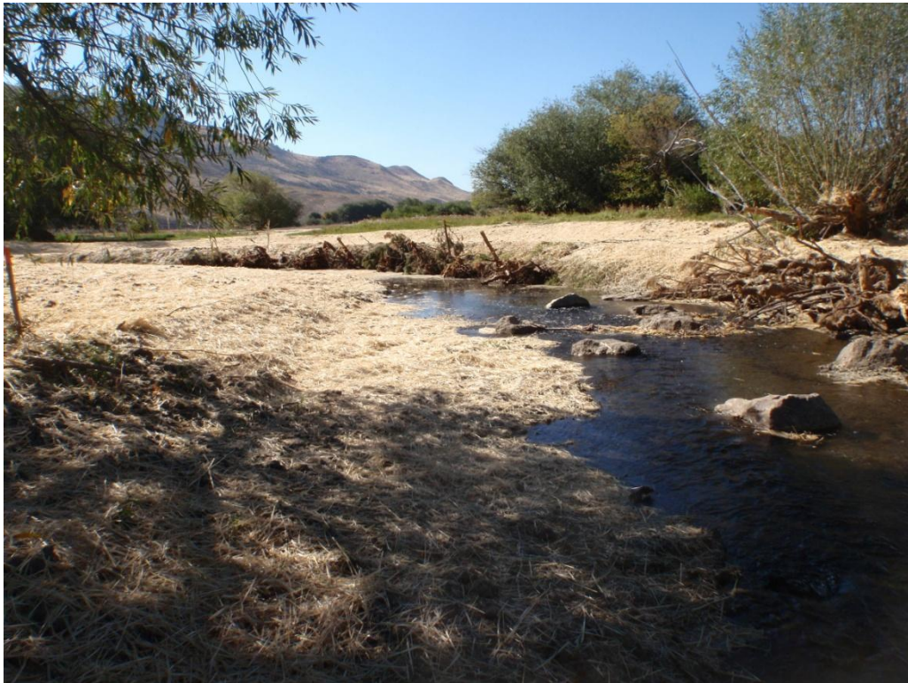
Photo 11. Excavated and re-sloped (3:1) vertical banks and widened floodplain. In-stream boulders, large wood structures, racking materials, and sedge mat placement. Banks were re-seeded, mulched, and planted with whips, container plants and protected with panel pods.
