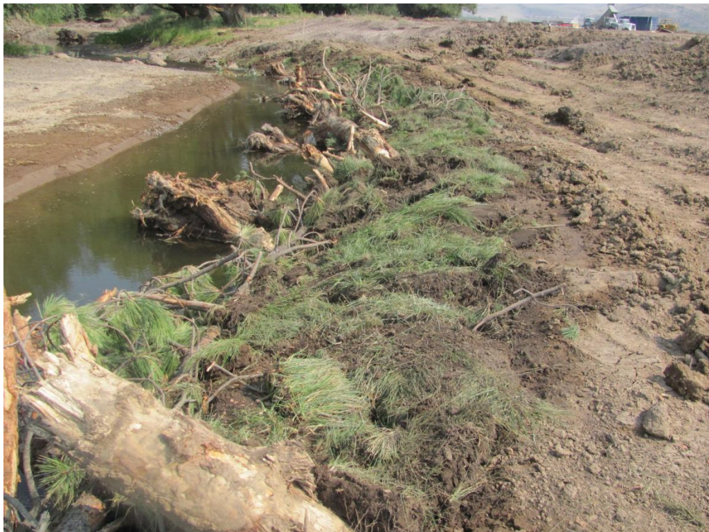
Photo 14. Excavated and re-sloped (3:1) vertical banks and widened floodplain. Large wood structures, racking materials, and sedge mat placement. Banks were mulched, re-seeded, and planted with whips, container plants, and protected with panel pods.
