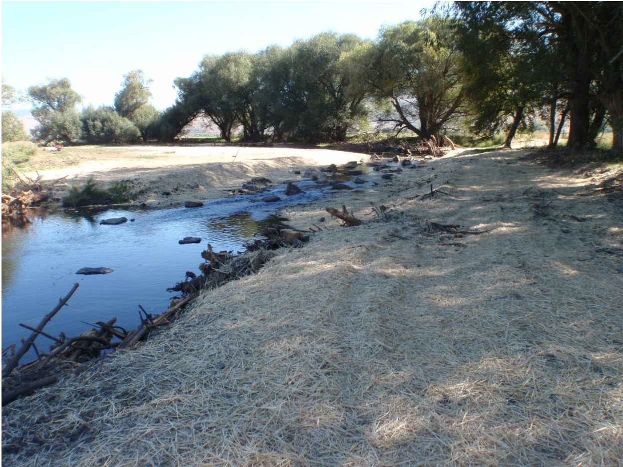
Photo 1: Completed Boulder, Large Wood Structure, Racking Materials, Sedge Mat Placement, Excavated Floodplain and Activated Old Meander Channel to become Main Stream Channel again, Preserve Old Meander Channel Existing Mature Trees, Re-seeded, Mulched, and Replanted with Willow Whips, Container Plants, and Protected with Panel Pods all Disturbed Riparian Areas.
