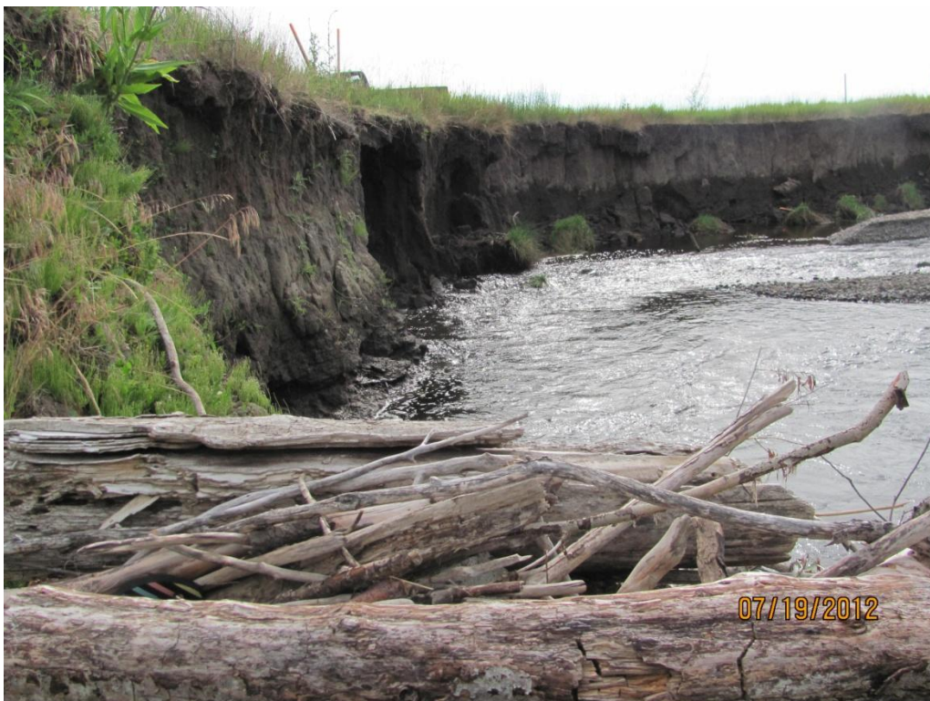
Photo 2. Vertical banks, pre-construction.
