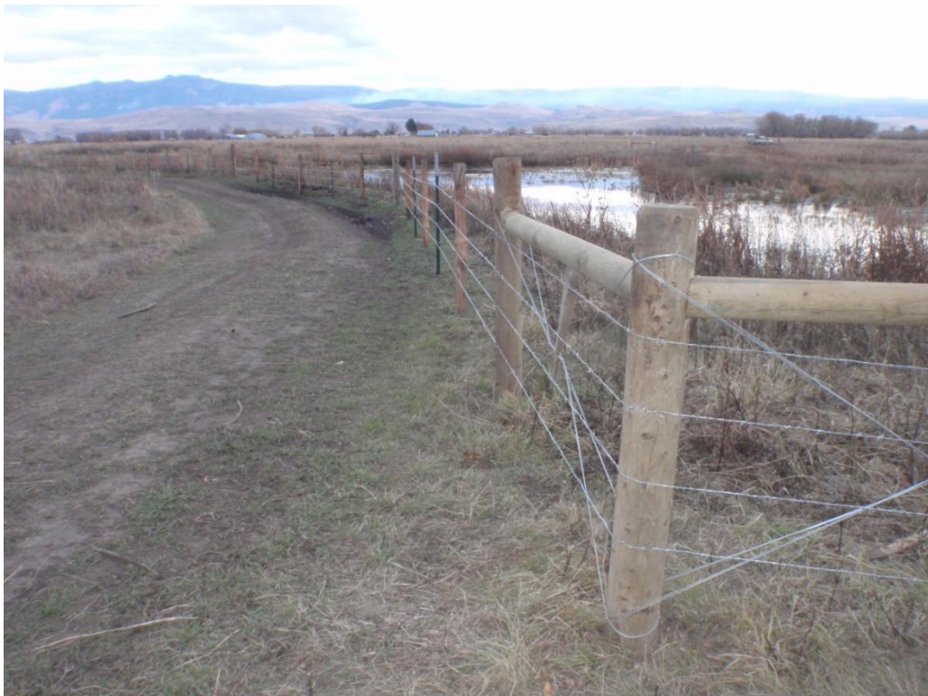
Photo 24. 15 year enclosure fencing protecting wetland area.
