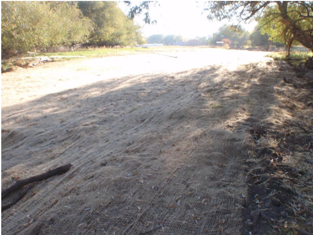
Photo 17. High water alcove with erosion control blanket, re-seeded, mulched, re-planted with whips, container plants, and protected with panel pods.
