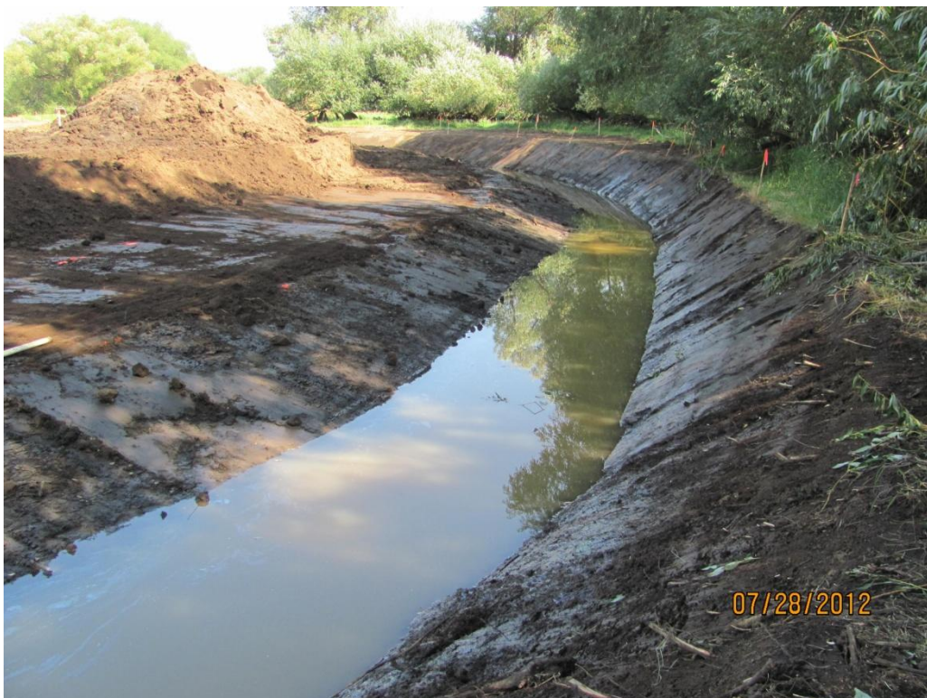
Photo 6. Excavation of new meander.
