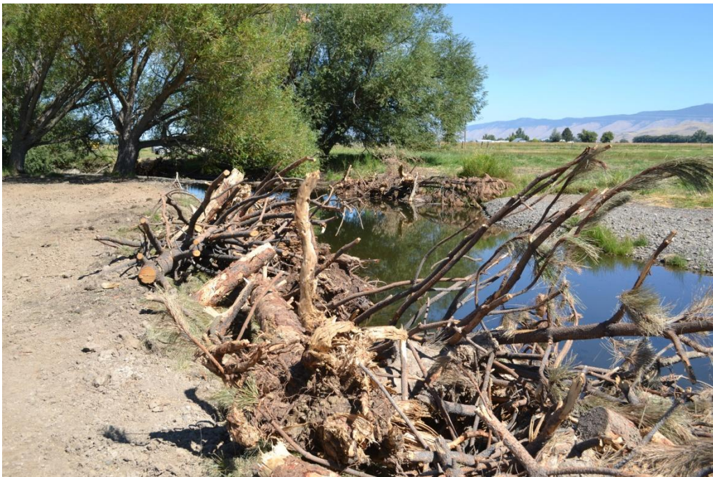
Photo 16. Excavated and re-sloped (3:1) vertical banks and widened floodplain. Large wood structures, racking materials, and sedge mat placement. Banks were mulched, re-seeded, and planted with whips, container plants, and protected with panel pods.
