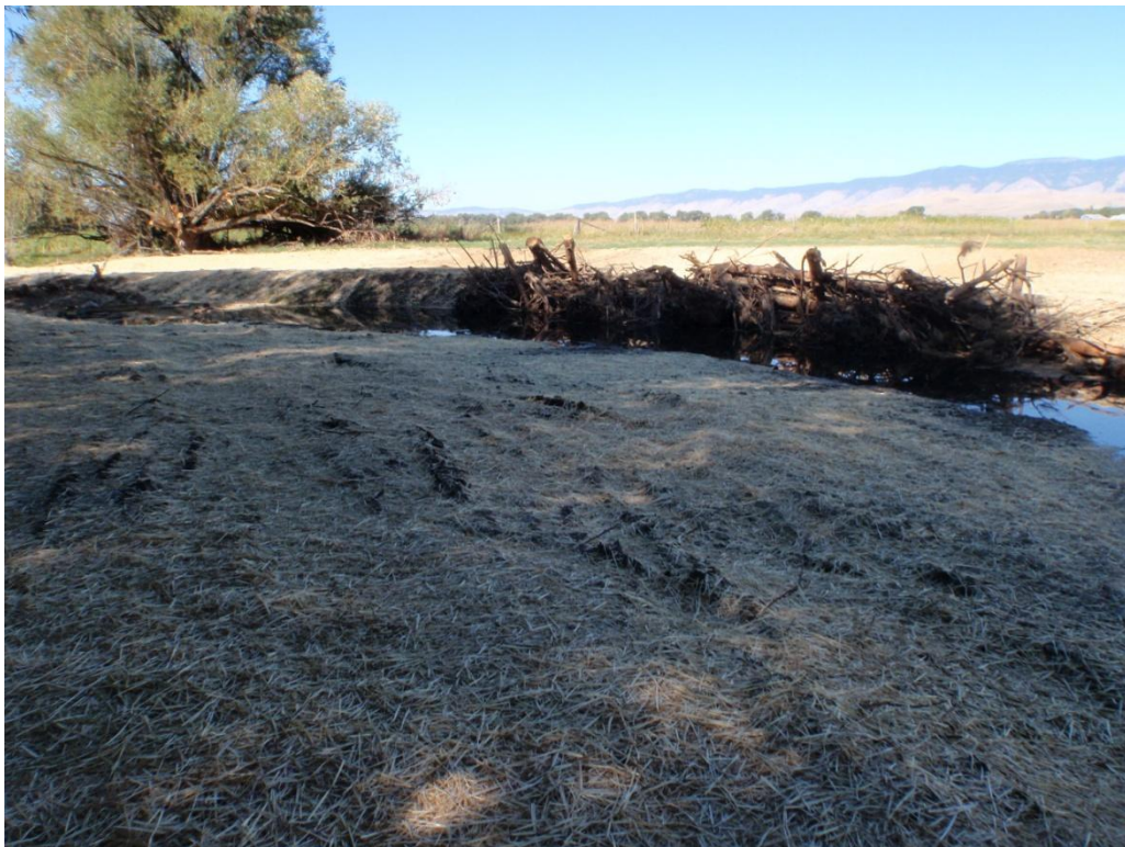
Photo 10. New meander. Excavated and re-sloped (3:1) vertical banks and widened floodplain. Large wood structures and racking materials placement. Banks were re-seeded, mulched, and planted with whips, container plants, and protected with panel pods.
