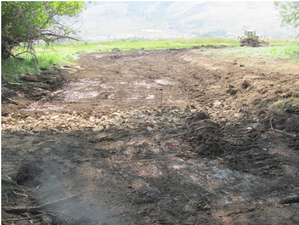
Photo 4. Completed upper side channel with entrance rock sill for sediment and flow control.
