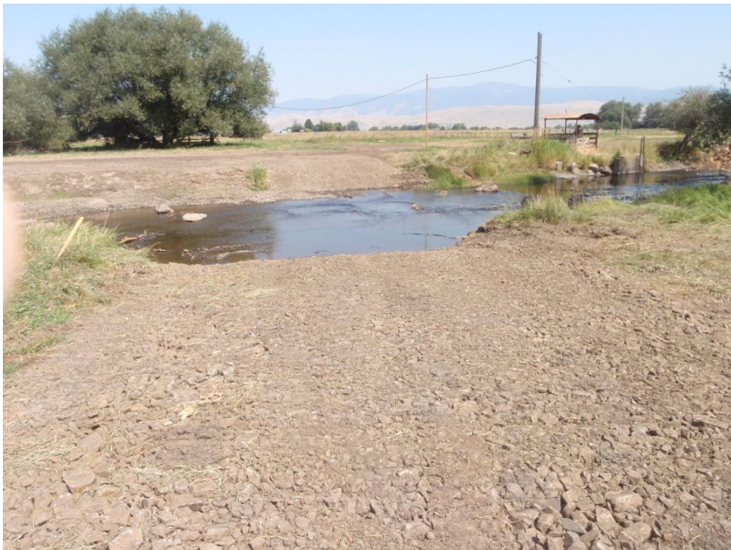
Photo 22. Completed hardened water crossing.
