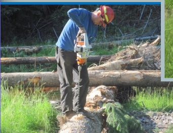
Logs were drilled at intersections and pinned with rebar.
