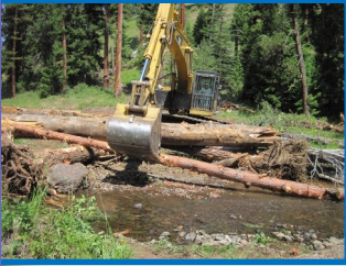
Excavators were used for building structures from large woody debris.
