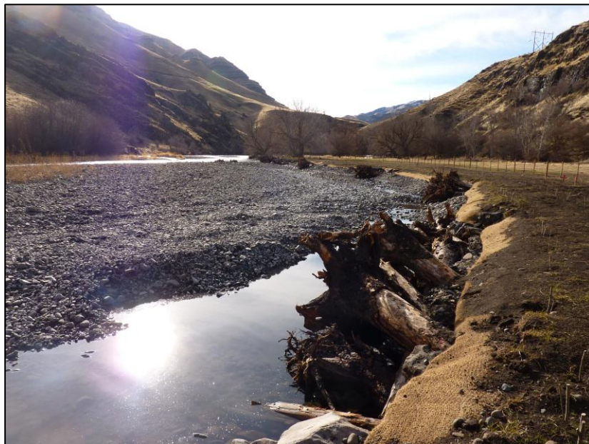
Photo 3: Photo taken on January 20, 2012. Bank has been shaped and covered with geo textile. Large woody debris features have been installed to provide aquatic habitat and maintain a stable stream bank. This side channel will be connected to the Imnaha main channel during the high flow months.
