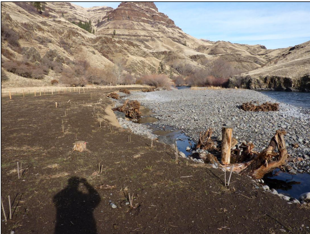
Photo 7: Post project photo looking downstream from the top of project. 5 wood features were installed that will significantly increase habitat conditions. Over time the riparian area will mature and over story vegetation will develop.
