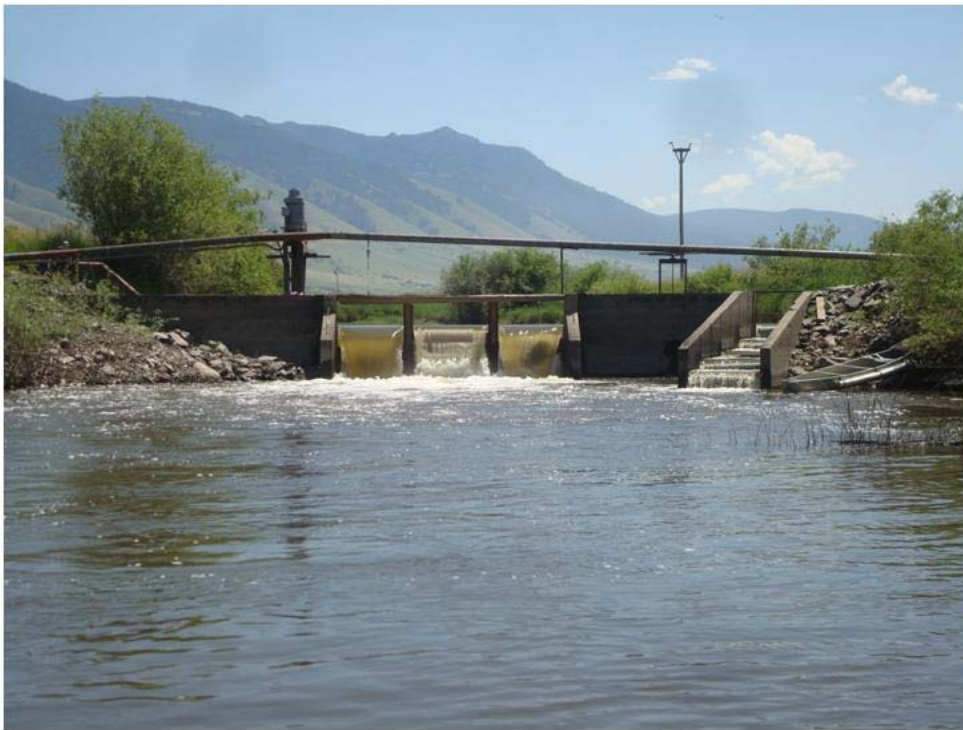
Figure 25. View looking upstream at Elmer Dam located at RM 13.1 used for irrigation water storage and diversion – Catherine Creek, Grande Ronde Subbasin. (Reclamation photograph by D. Stelma – July 9, 2010).
